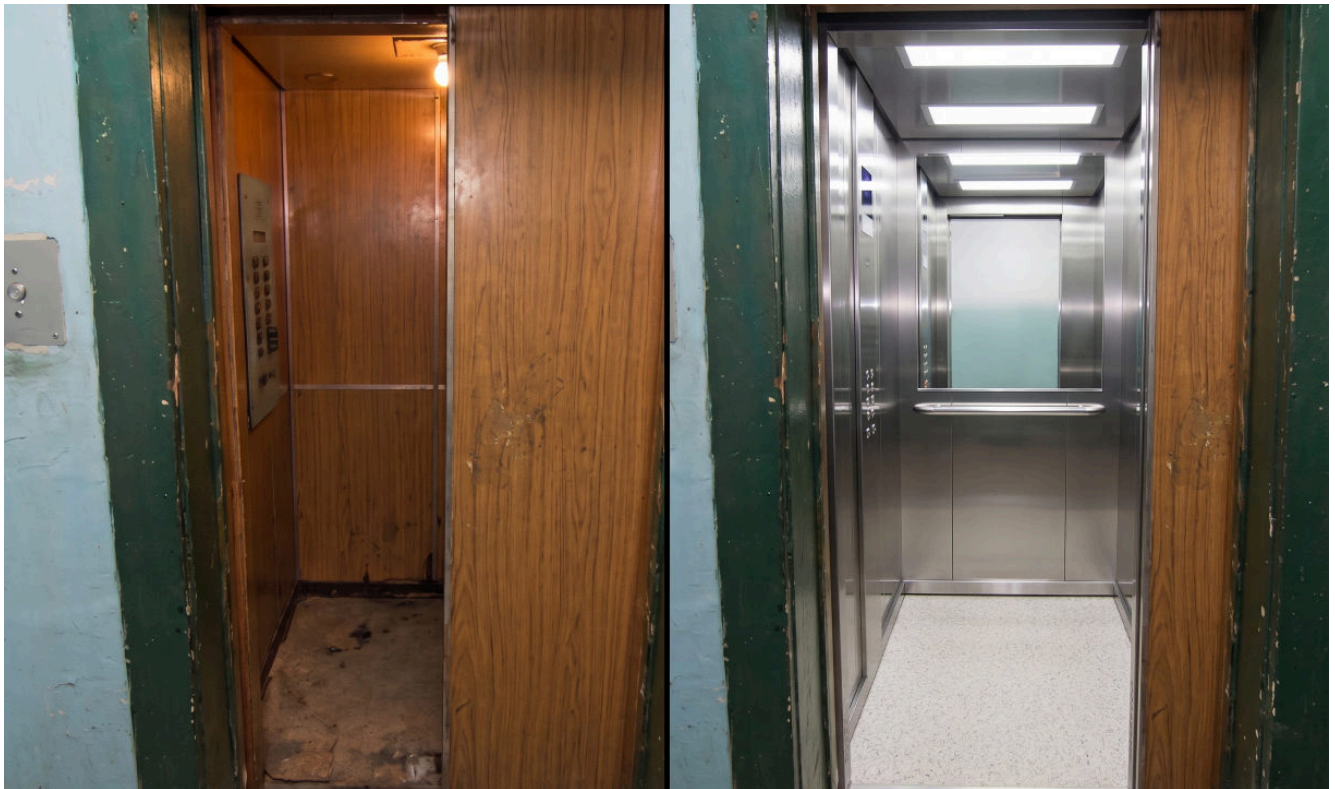
The same shaft, the same building: on the left the old lift before replacement, on the right the new one after.
